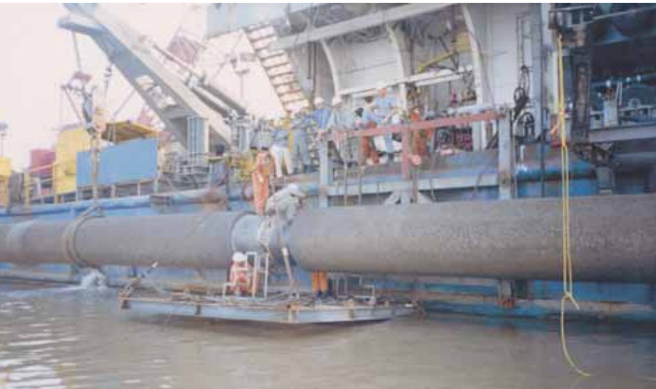
↑ Tie-in of submarine pipes and lowering. (Pipe lay barge in background)
