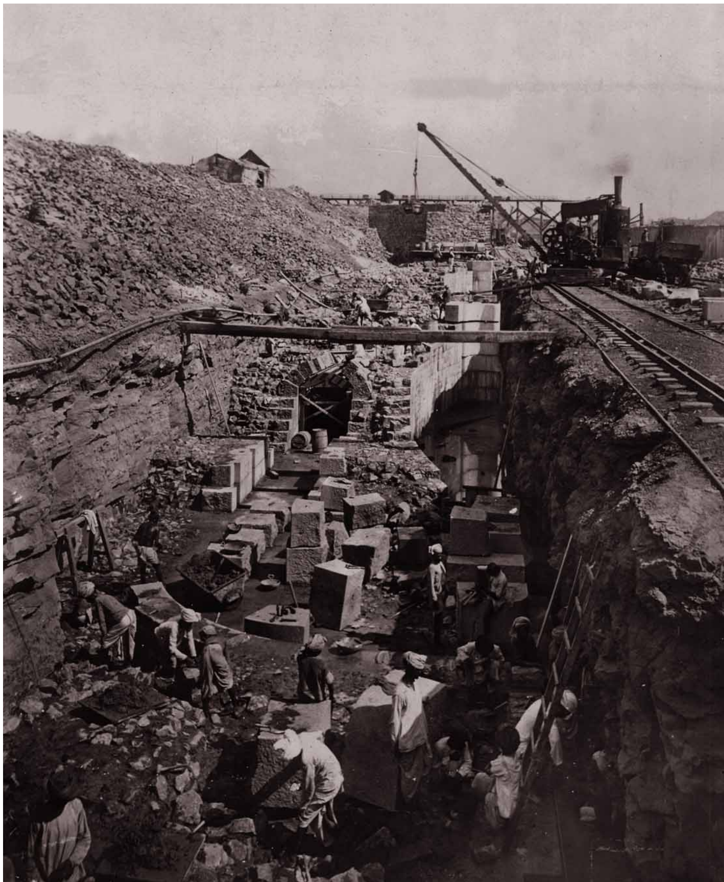
Construction work seemed to be never ending in the first quarter of the 20th century. Picture shows Hughes Dry Dock under construction (19 April 1910).
