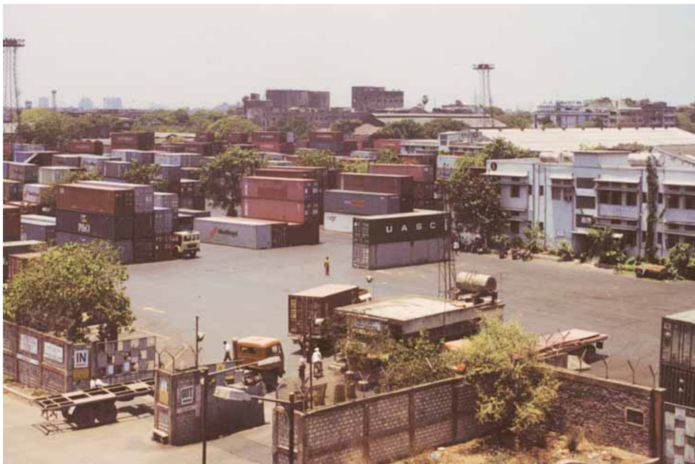
View of Container Freight Station, Sewree.
