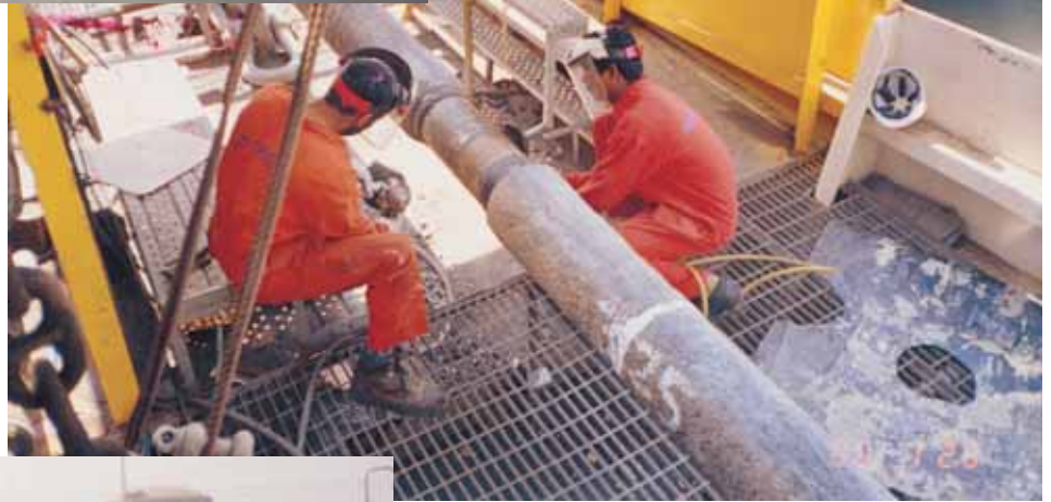
↑ Joining of Submarine pipe sections on the pipe lay barge.
