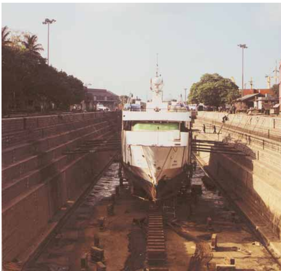
O.N.G.C. Vessel in the Merewether Dry Dock.
