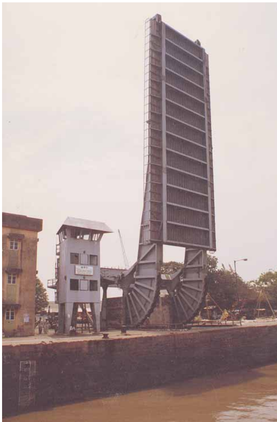
The Rim Bascal Bridge, which spans the entrance lock in the Indira Dock, consists of a single leaf with a clear span of 100 ft and carries a 24 ft wide carriage way.
