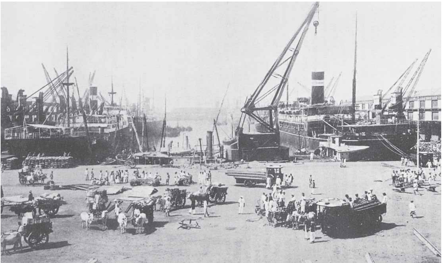
Shipping at the West and Jetty Wharves, Alexandra Dock, with the Port Trust 60-ton floating crane at work (1925).
