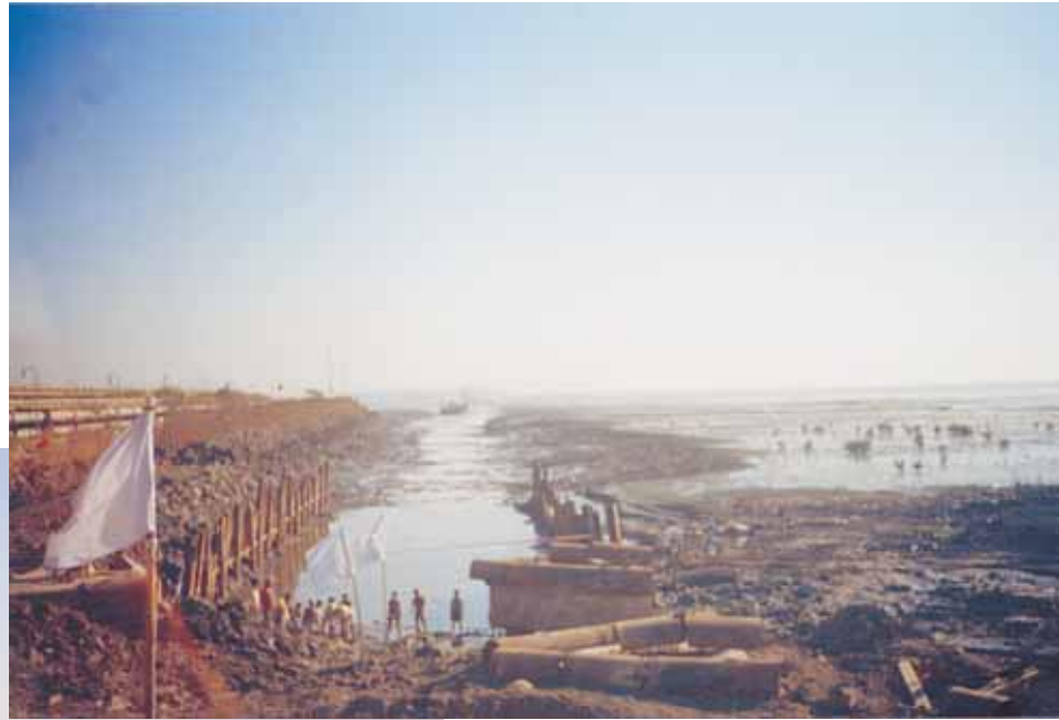
↑ A view from Pir Pau landfall point.
