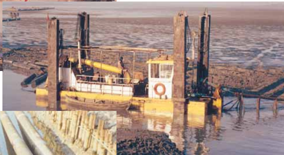
↓ Dredger a closure view
