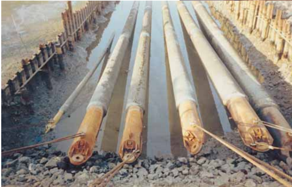
Six Submarine pipelines as they approach ↓ Jawahar Dweep shore
