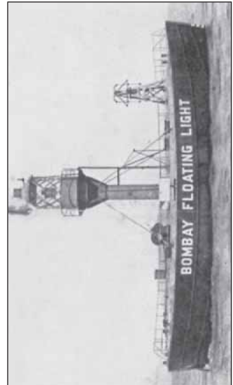
BOMBAY FLOATING LIGHT Built by Messrs Barbier, Benard and Turenne at Nantes, France in 1929. Length o.a. 70'-0"; Breadth 27'-0"; Depth 13'-6"; Draught 7'-6" Height from water to focal plane of light 32'-0" Light equipment consists of a White light of 1560 candle-power giving a triple flash, plus 1 sec. flash, plus 25 secs. dark, plus 1 sec. flash, plus 17 secs. dark, to operate uninterruptedly for 12 months. Visibility 15 miles in clear weather. Fitted with Sun valve which extinguishes the light during daylight and causes it to reappear when daylight fails.
