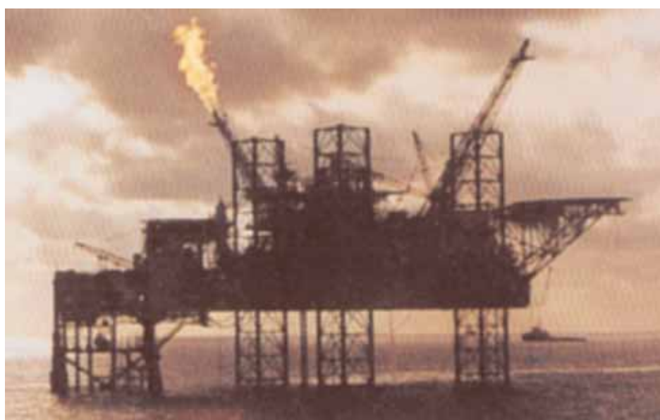
Panna & Mukta — off Bombay High. Crude Oil Natural Gas platform-Northwest of Mumbai.
