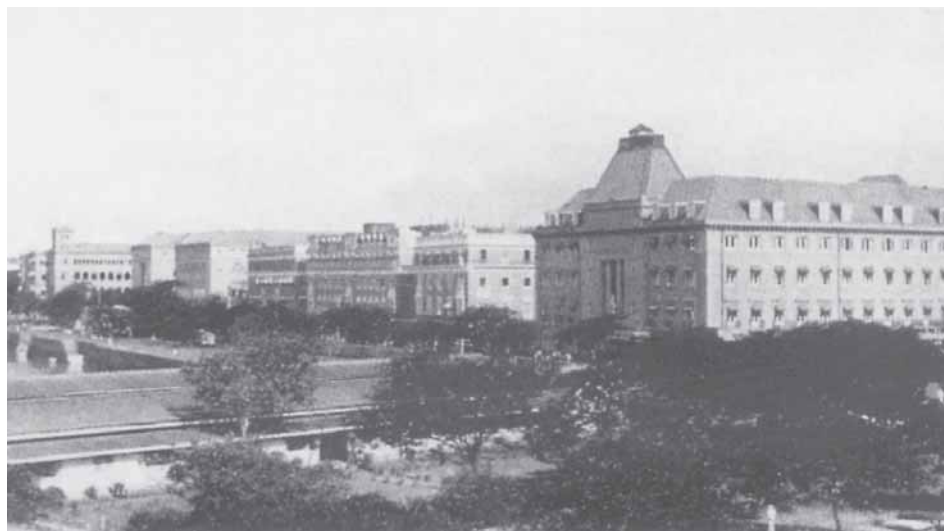
Ballard Estate, with the P&O and BISN Co's offices in the foreground.
