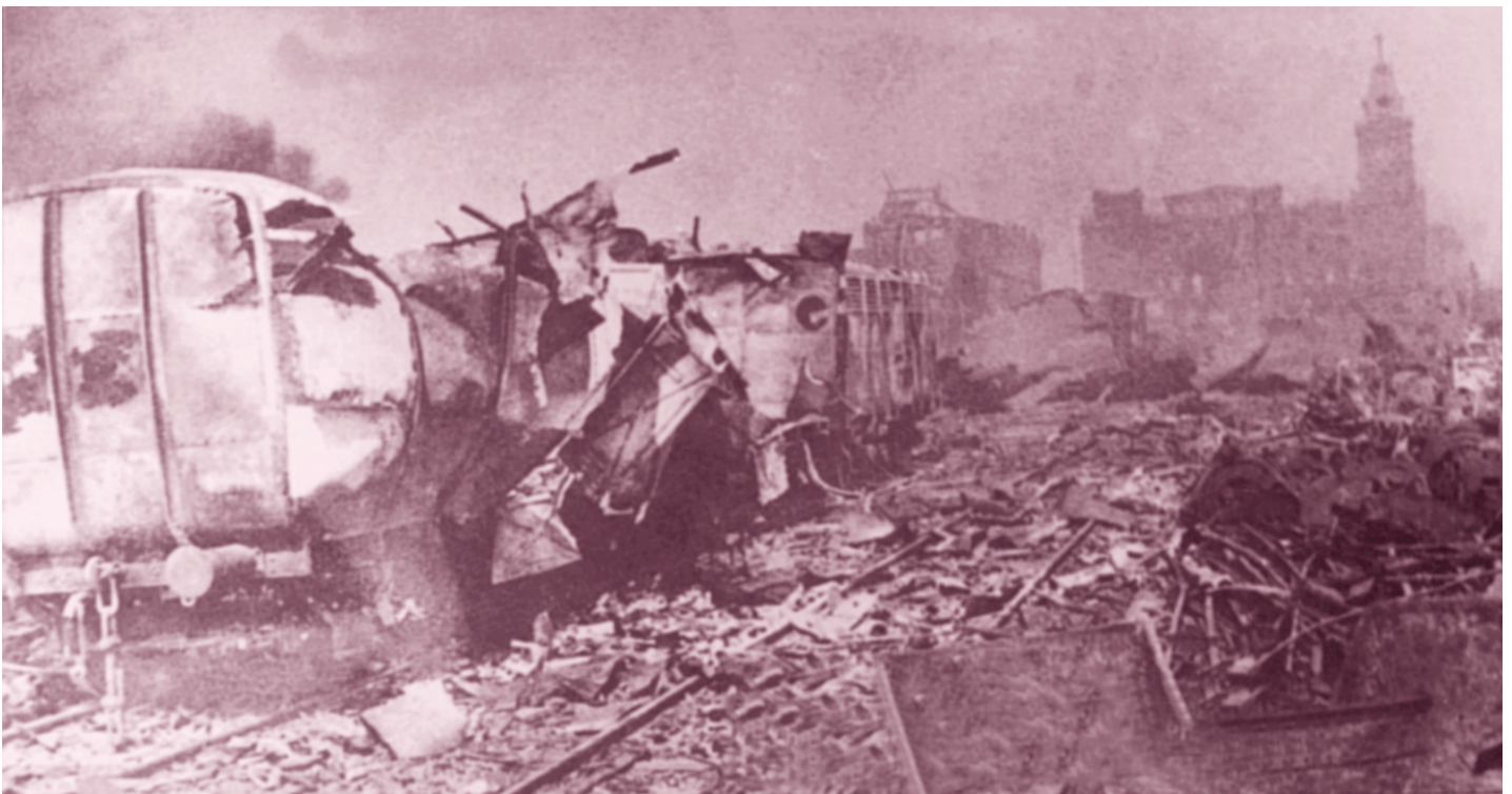
The BPT railway suffered severe damage, as did the GIP. In the background is the Prince's Dock building, the Ghadial Ghodi (April 1944).
