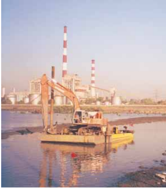
↓ Pre trenching in progress at Pir Pau end.
