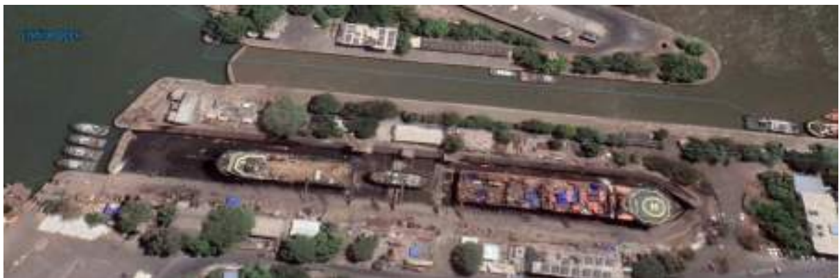
Figure 2.38 View of Dry Dock with Three Vessels Docked
