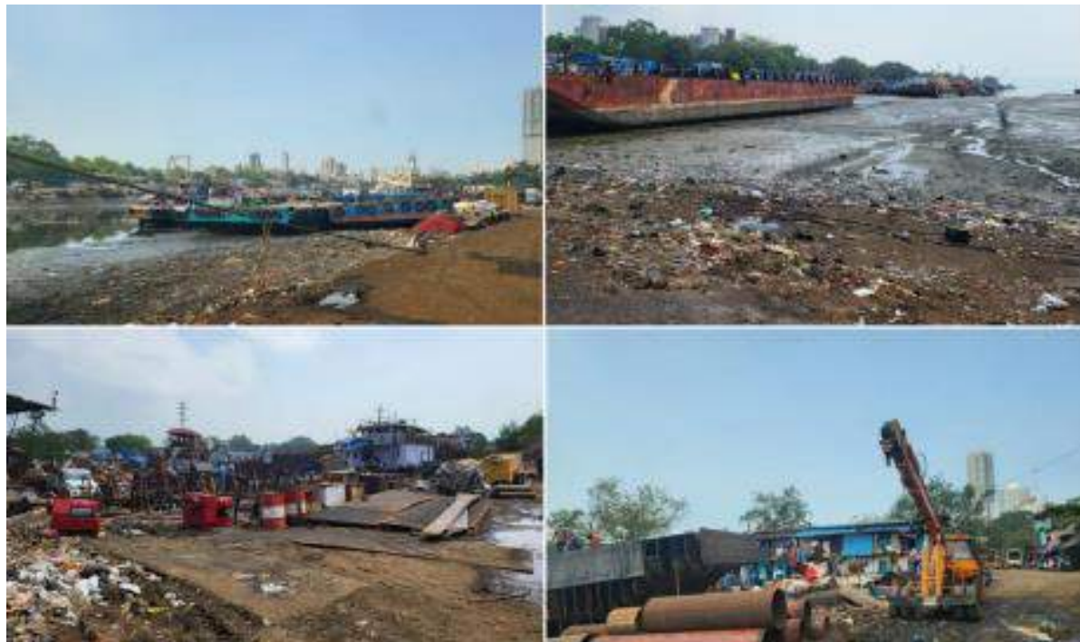
Figure 2.35 Existing Ship Repairs at Bunders – I
