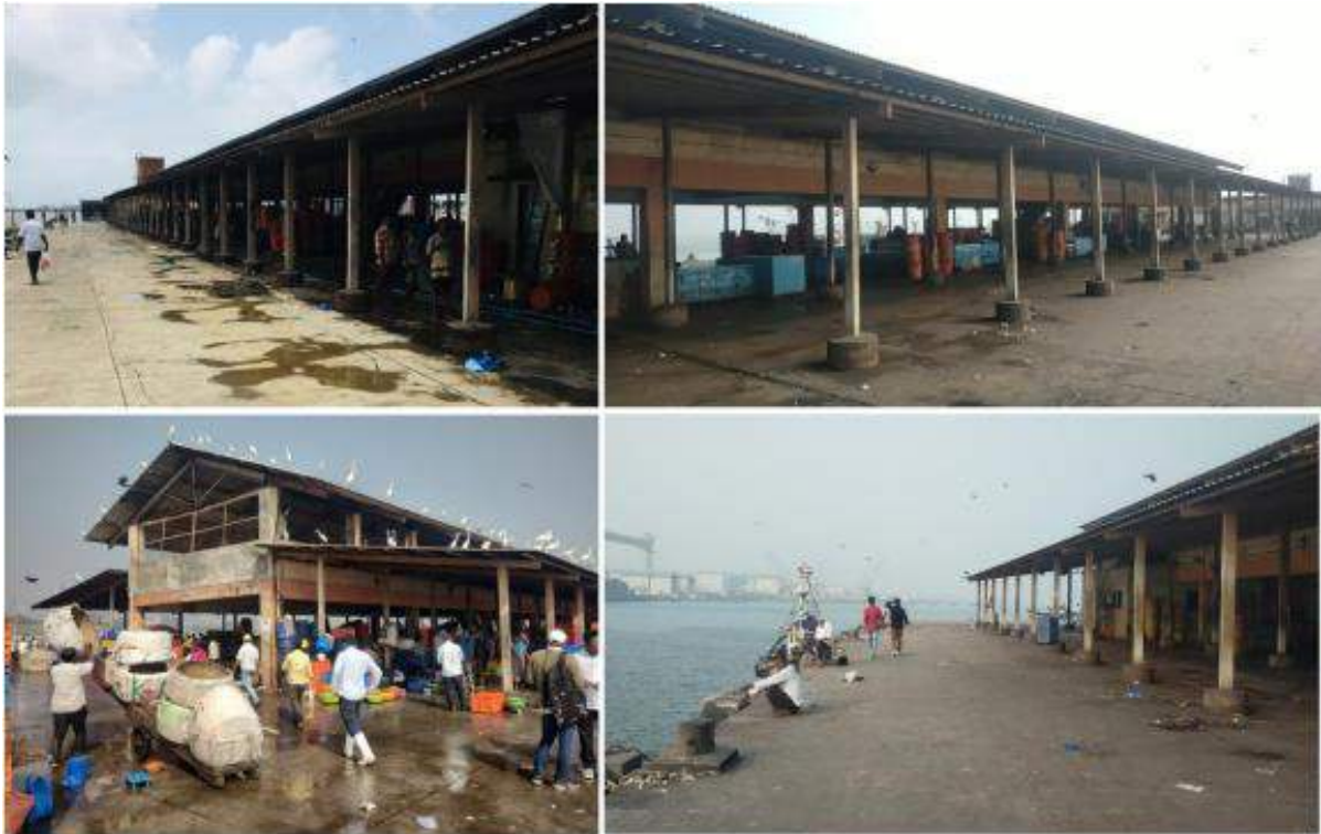
Figure 2.44 Ferry Wharf Berthing Area
