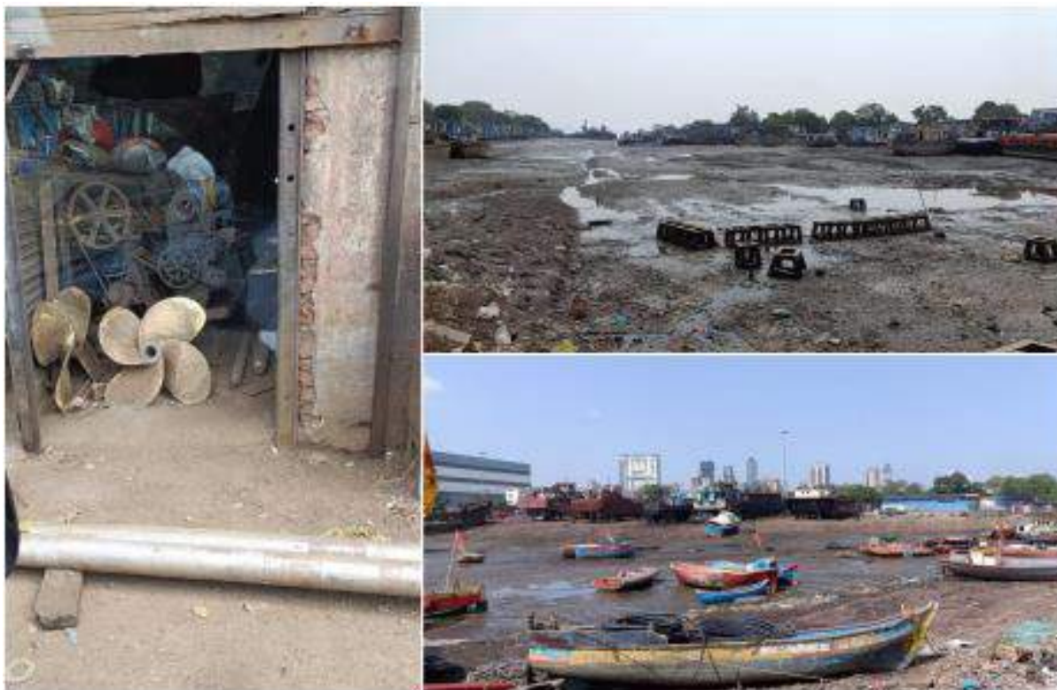
Figure 2.34 Existing Ship Repairs at Coal & Lakri Bunders
