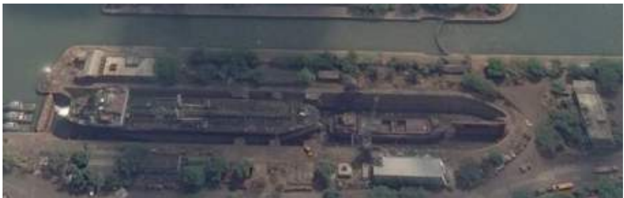
Figure 2.37 View of Dry Dock with Two Vessels Docked
