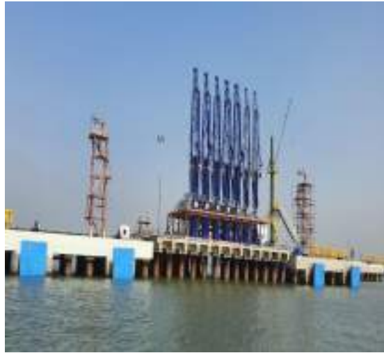
Figure 2.20 Fifth Oil Terminal at Jawahar Dweep
