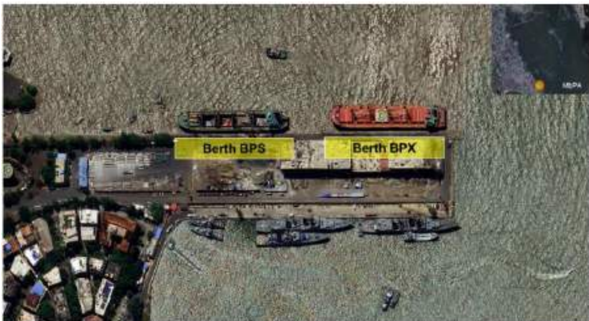
Figure 2.26 Berths at Ballard Pier (Source: Traffic Study Report prepared by CRISIL)
