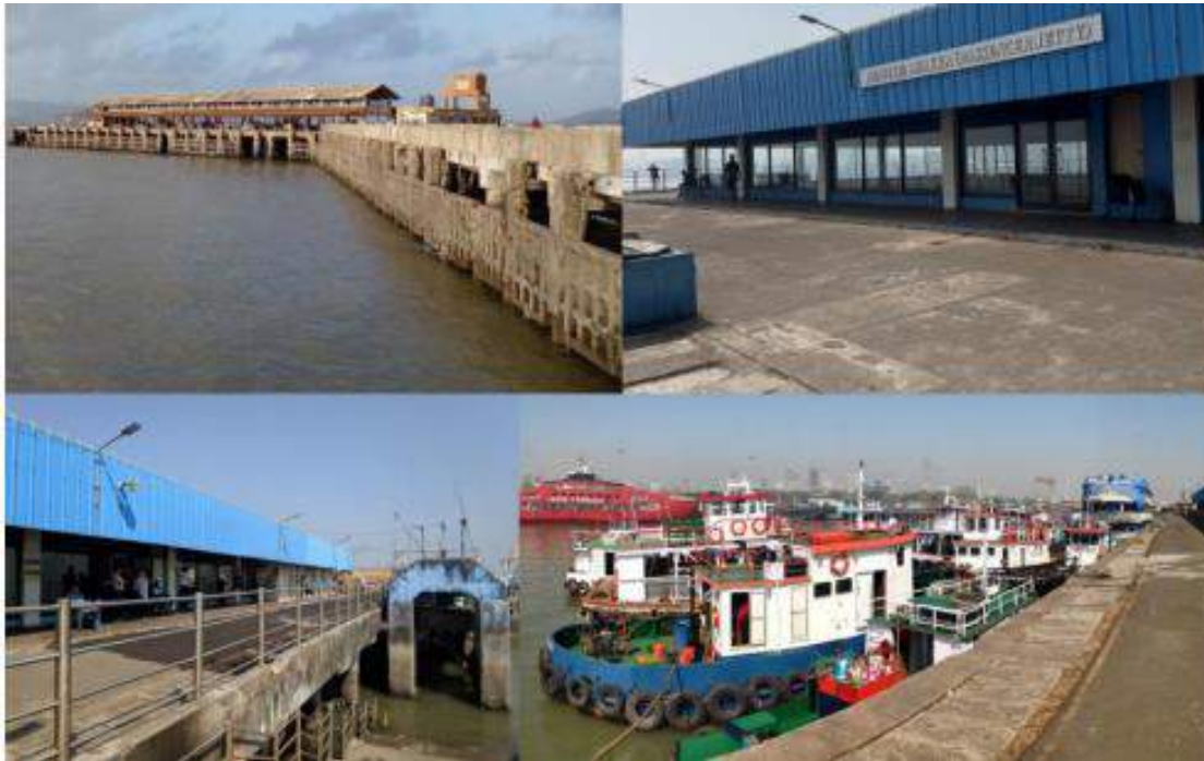
Figure 2.59 Vessel Berthing Infrastructure at Ferry Wharf
