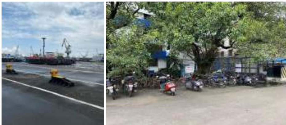
Figure 3.6 Open Storage/Operation Area at 1ID, 2ID, 3ID& Parking Lot near Blue Gate
