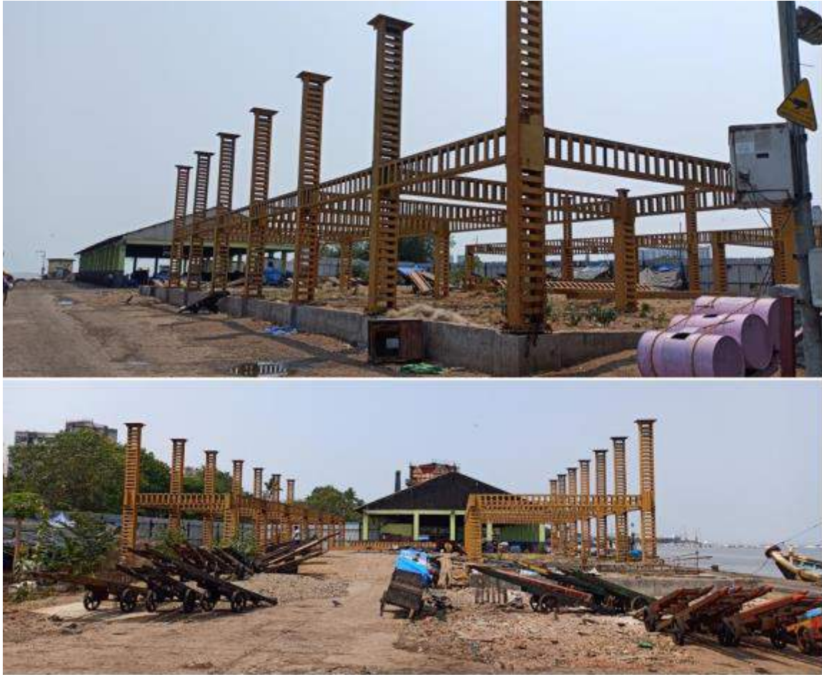
Figure 2.52 Under Construction Ice Plant at Sassoon Dock
