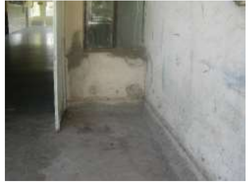
2 nd Floor Near Terrace - After
