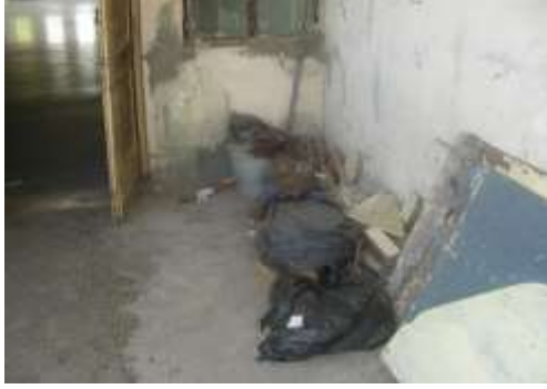
2 nd Floor Near Terrace – Before
