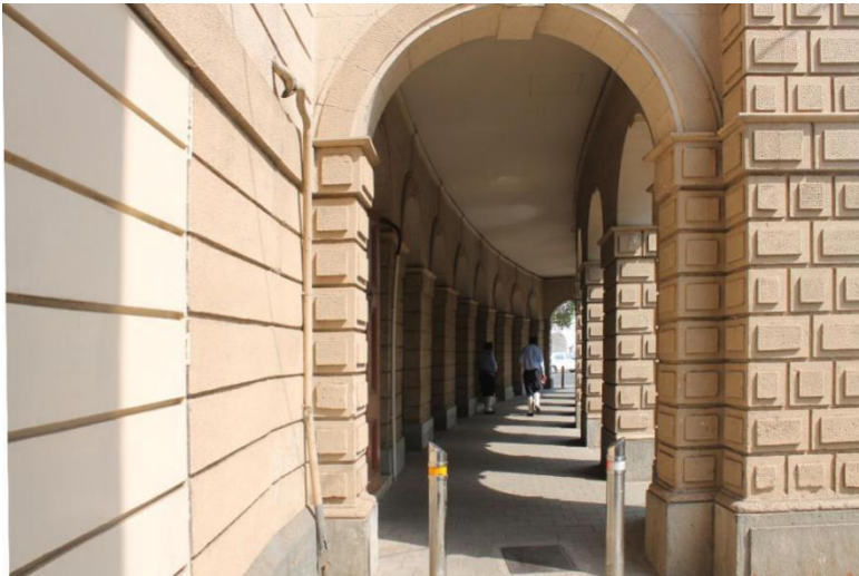
Image 3: Covered Arcade in Ballard Estate
