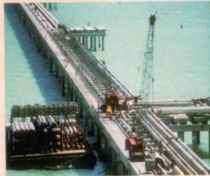
Third Chemical Berth
