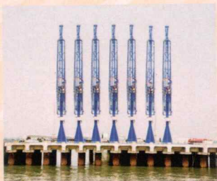
Fifth Oil Berth (Biggest Oil Terminal with capacity of 22 MMT)
